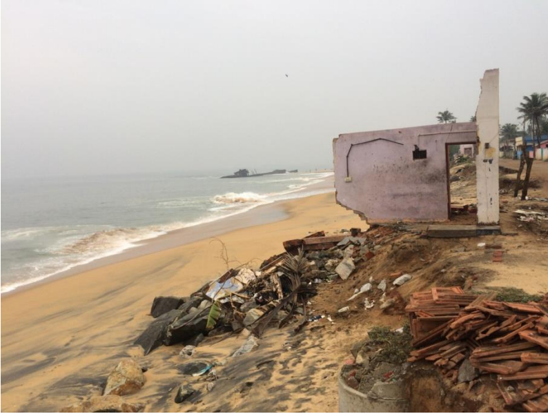
House damaged by Erosion in Eravipuram
