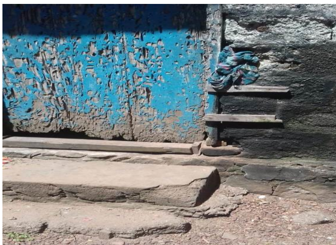
Condition of House
